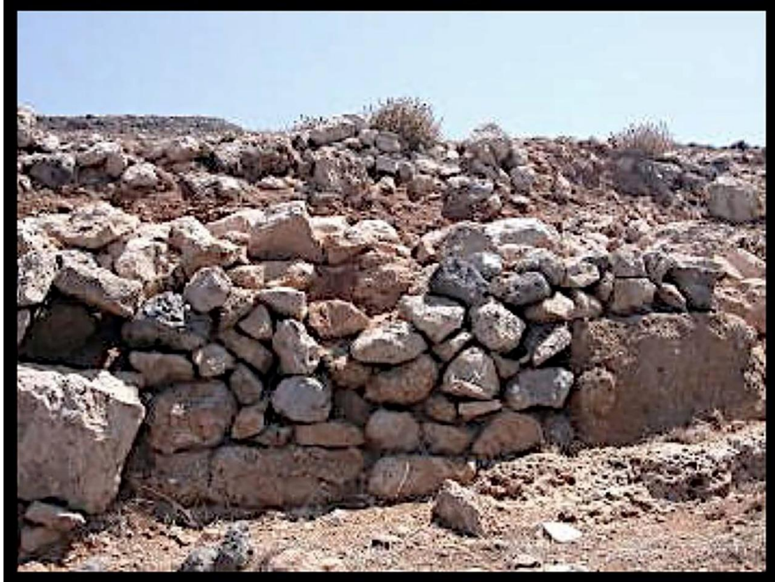
Fig. 5 A part of the western fortification wall destroyed and repaired.
